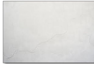
Hairline Cracks
